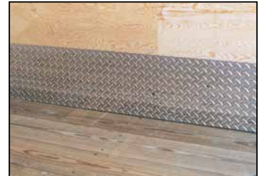
ATP Wall Guard and 1 1/2" T & G Flooring
