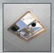
Roof Vent with Exhaust Fan
